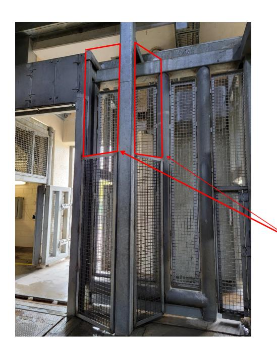
INSTALL NEW GALV. STEEL MESH PANELS BETWEEN COLUMNS (MATCH EXISTING) 50X50X12GA MESH, WELDED AT ALL JOINTS & TO ALL STEEL BARS/COLUMNS W/ 50X8 GALV. FLAT BAR WELDED ON EDGES OF MESH. (TYP)
