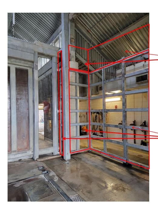
INSTALL NEW 4' HIGH GALV. STEEL MESH PANELS ABOVE EXISTING WALL (MATCH EXISTING) 50X50X12GA MESH, WELDED AT ALL JOINTS W/ 50X8 GALV. FLAT BAR WELDED ON EDGES OF MESH. (TYP) ATTACH TO BOTTOM WALL W/ WELDED STANDOFFS. REINFORCE AS REQUIRED.
