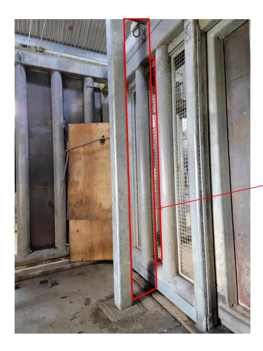
INSTALL NEW GALV. STEEL MESH PANELS BETWEEN COLUMN AND WALL (MATCH EXISTING) 50X50X12GA MESH, WELDED AT ALL JOINTS & TO ALL STEEL BARS/COLUMNS W/ 50X8 GALV. FLAT BAR WELDED ON EDGES OF MESH. (TYP)
