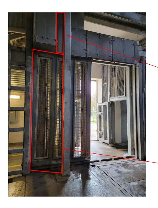
INSTALL NEW GALV. STEEL MESH PANELS BETWEEN COLUMN AND SERVICE DOORS (MATCH EXISTING)
